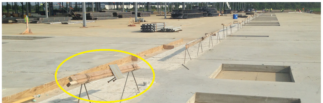
Rebar "bump" cap (also known as "mushroom cap"). Not used for impalement protection.
